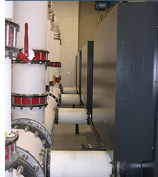
Above image shows an ample sized header with insulation to limit heat transfer to the package cooling air.
